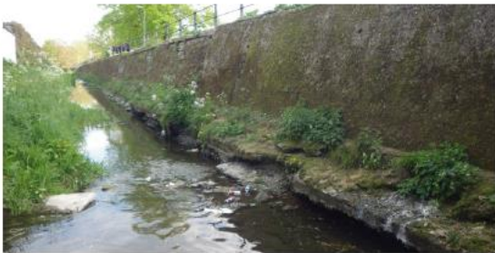
Existing concrete wall on south bank of Turkey Brook
